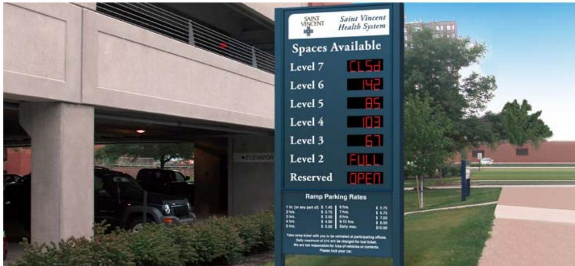
Dynamic wayfinding signs are an effective method to improve the parking experience for drivers searching for a parking space in a parking facility with multiple levels, or many lots spaced closely together. Drivers are able to see the real-time parking vacancies, and can go where the most parking is available to find a space. The Dynamic wayfinding signs are ideally followed up with additional static directional signage at critical junctions to provide users with further directional information.
