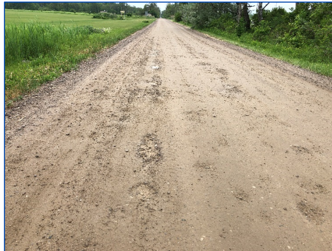
Figure 4.10: Potholes, Loose Gravel and Breakups – Toll Road (Section No. 345)
