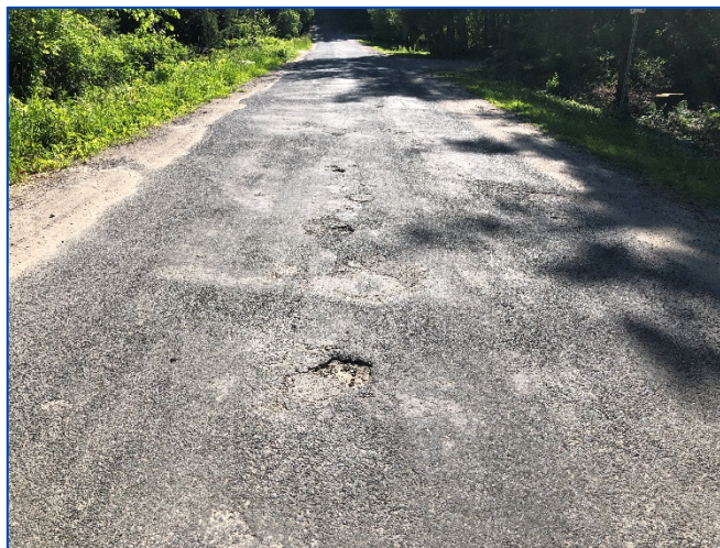
Figure 4.7: Ravelling and Aggregate Loss, Potholes – 16 th Sideroad between Bathurst Street and West End (Section No. 21)
