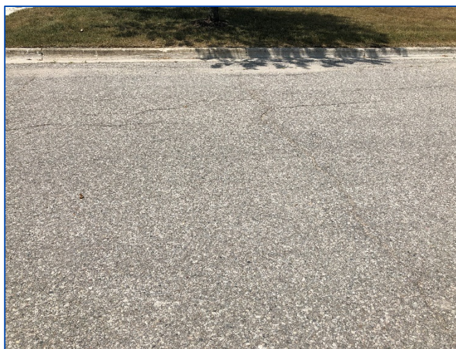
Figure 4.1: Moderate Ravelling – Russell Snider Drive, Nobleton (Section No. 2116)
