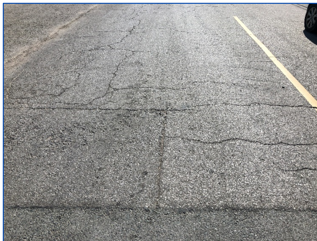
Figure 4.3: Longitudinal and Transverse Cracking – Old King Road, Nobleton (Section No. 2000)
