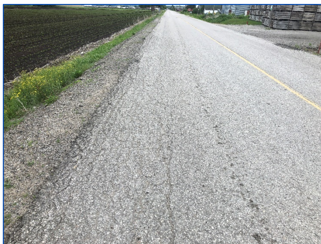
Figure 4.4: Pavement Edge Cracking – Strawberry Lane (Section No. 307)
