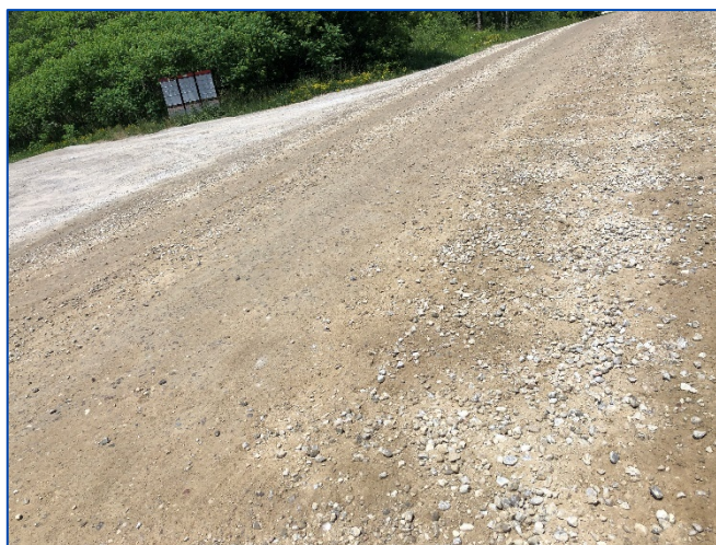
Figure 4.11: Washboard and Rutting – Concession Road 7 (Section No. 233)
