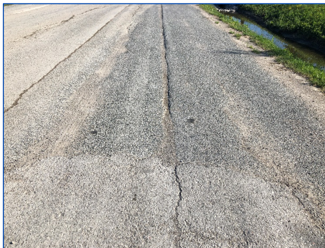
Figure 4.2: Wheel-Track Rutting – Magnum Drive, Schomberg (Section No. 3002)
