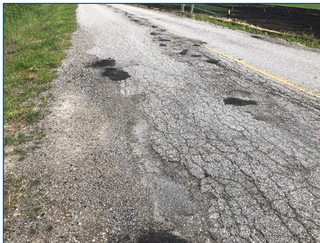
Figure 4.9: Alligator Cracking on Surface-Treated – Wist Road (Section No. 287)
