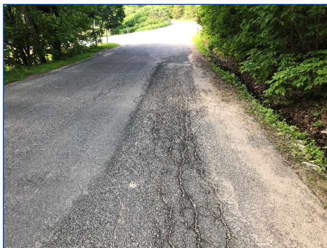
Figure 4.8: Surface-Treated Pavement Distortion – Lorne Avenue, Kettleby (Section No. 109)
