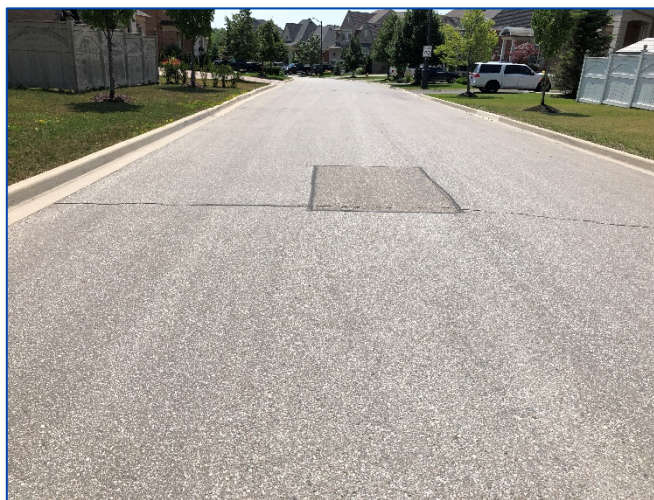
Figure 4.6: Pavement Patch – Blue Beech Trail, Nobleton (Section No. 2137)
