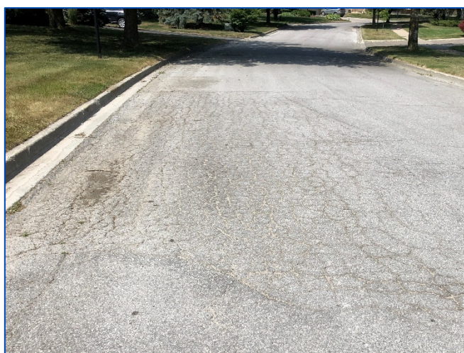
Figure 4.5: Alligator Cracking – Robb Drive, Nobleton (Section No. 2084)
