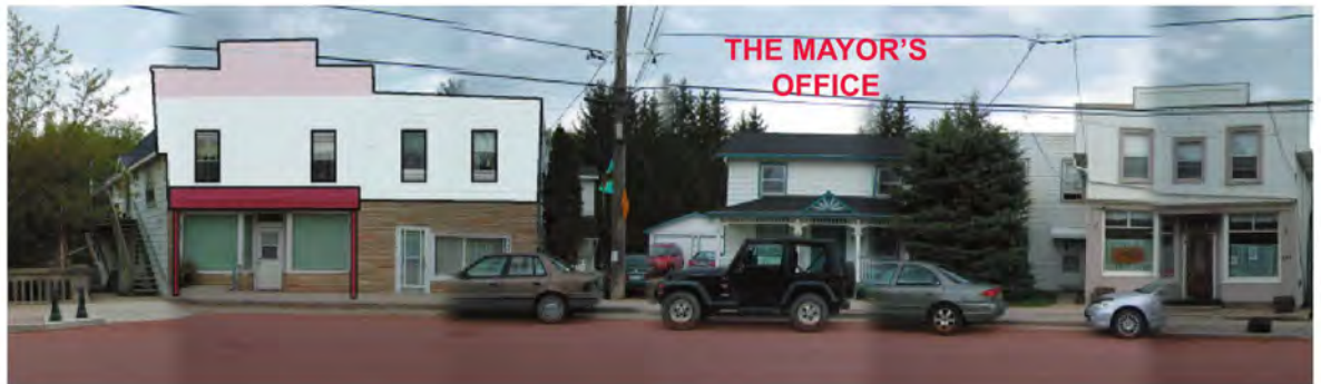
Figure 6.13 -West Side of Main Street - South of Schomberg River (continued from above)
