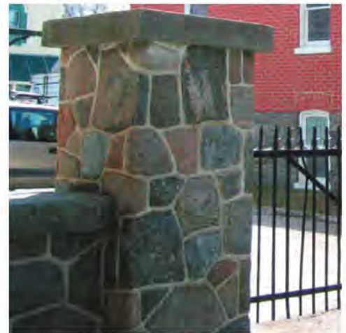
Figure 4.28 The existing stone wall on Main Street at the entrance to the Fairgrounds. A more durable natural stone retaining wall product should be used to maintain the look and feel of the original wall for when it needs to be replaced.
