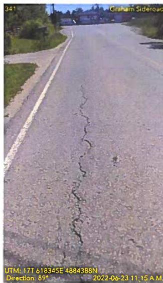
Figure 15: Mid-lane Cracking Example
