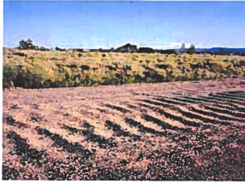
Figure 21: Washboarding Example (Photo from King Not Available)
