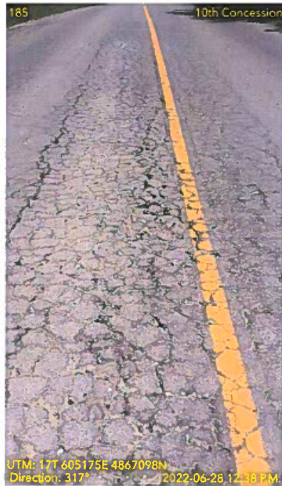
Figure 10: Centreline Alligator Cracking Example
