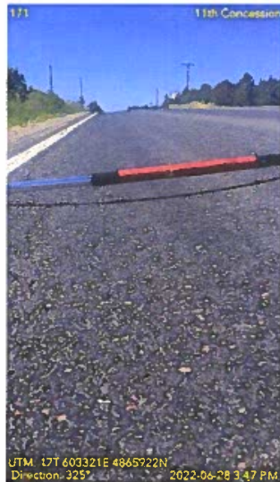
Figure 5: Wheel Track Rutting Example
