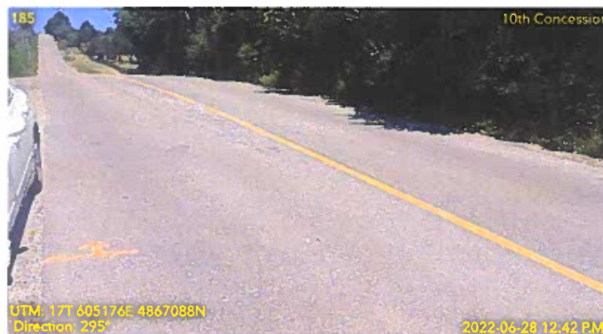
Figure 2: Ravelling and Aggregate Loss Example
