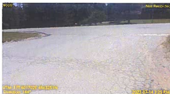
Figure 14: Transverse Alligator Cracking Example
