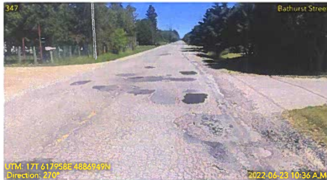
Figure 16: Potholing and Patching Example
