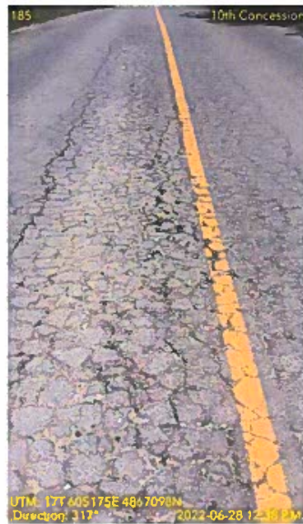
Figure 8: Wheel Track Alligator Cracking Example
