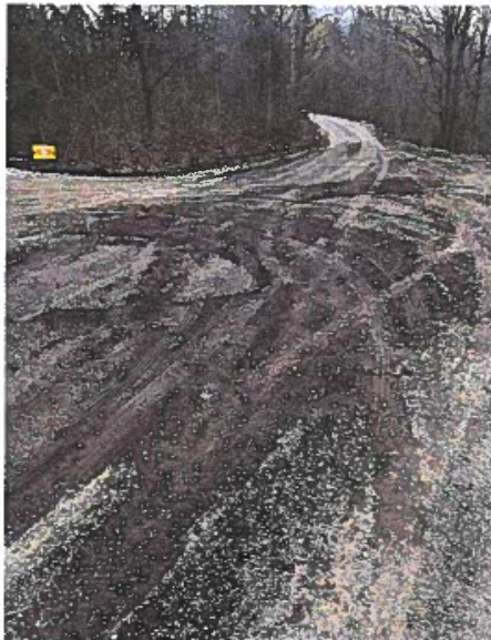
Figure 18: Soft Spot Example
