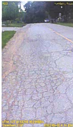
Figure 12: Pavement Edge Alligator Cracking Example
