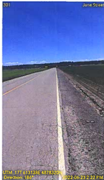
Figure 11: Pavement Edge Cracking Example
