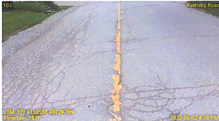
Figure 9: Centreline Cracking Example
