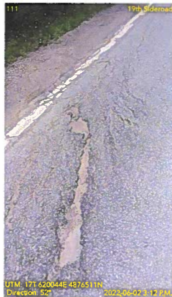
Figure 4: Rippling and Shoving Example
