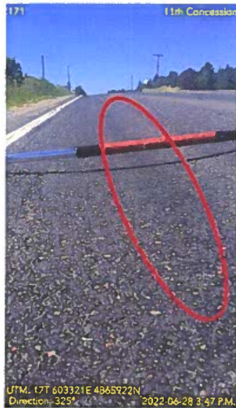
Figure 3: Flushing Example
