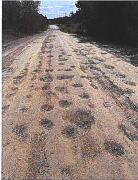
Figure 20: Potholing Example
