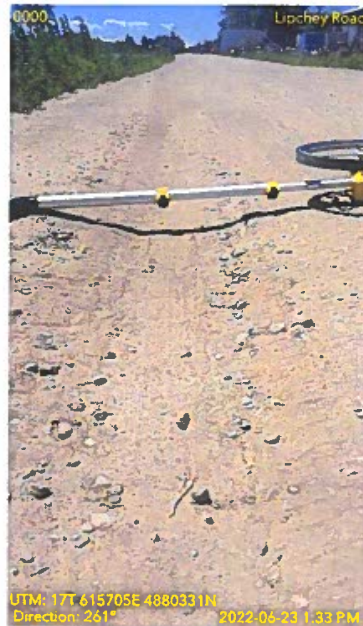
Figure 23: Rutting Example
