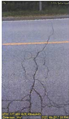
Distress 13: Transverse Cracking (Alligator)
