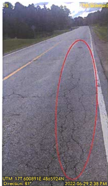
Figure 7: Wheel Track Cracking Example
