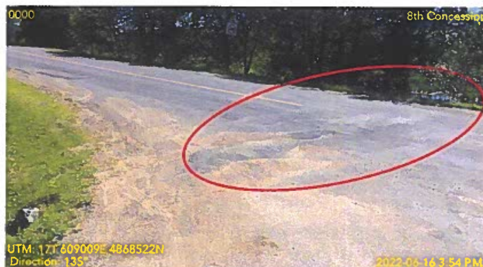
Figure 6: Distortion Example
