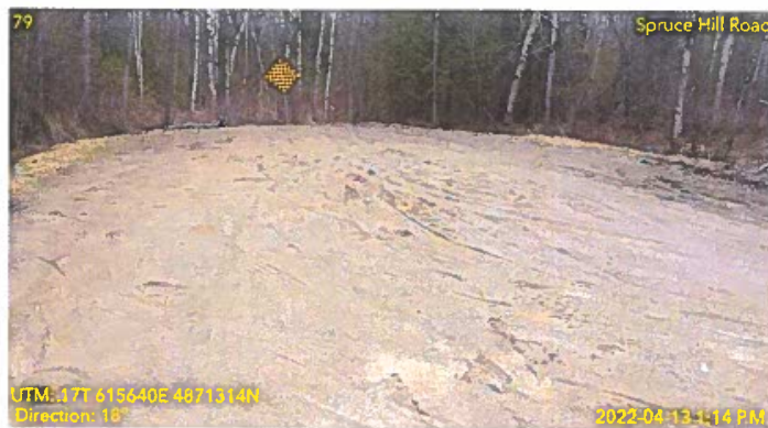
Figure 19: Spring Breakup Example
