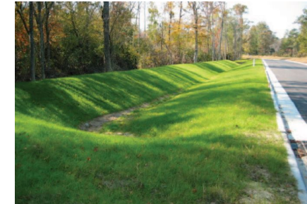
Grassed Swale located upstream of the facility
