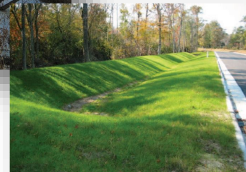
Grassed Swale located upstream of the facility
