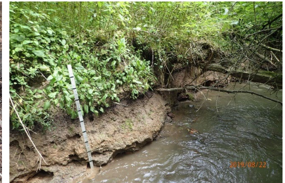
Channel Erosion identified during inspection of natural channels
