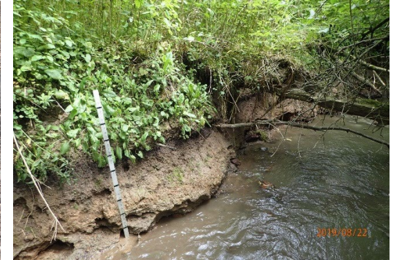
Channel Erosion identified during inspection of natural channels
