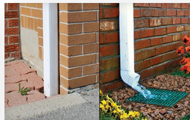
Downspout Disconnection
