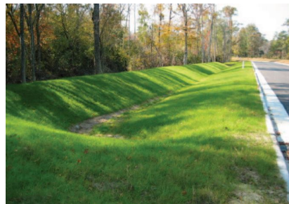
Grassed Swale located upstream of the facility
