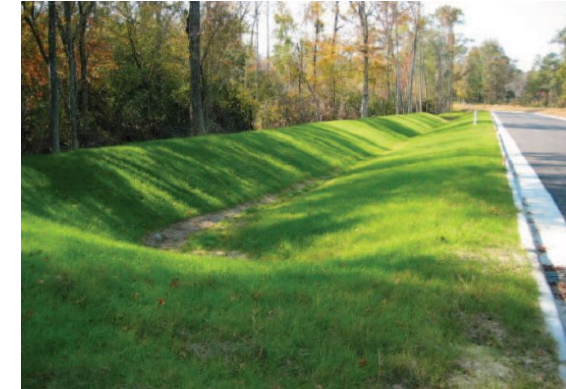
Grassed Swale located upstream of the facility
