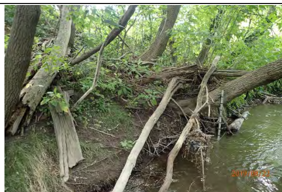
Leaning trees and exposed roots along the bank. Note the woody debris present along the banks and in the channel.
