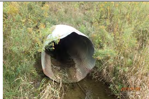
Photograph of the upstream CSP. Erosion was noted surrounding the CSP indicating the crossing may be undersized.
