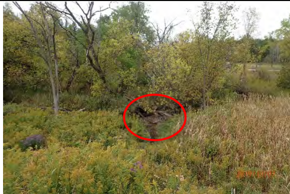
Photograph taken facing downstream of Lloydtown/Aurora Road. The confluence (circle) with a larger tributary was approximately 10 m downstream of the CSP.
