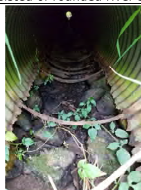
CSP at upstream extent of reach HN4-4 . Note the degradation of the pipe.
