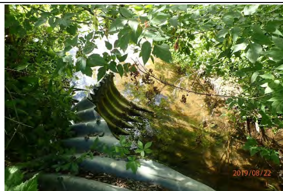
The CSP upstream of Centre Street was misaligned with channel creating a possible concern.
