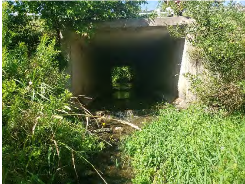
Photograph facing upstream at the downstream extent of the road crossing. Channel bed was lower than the box culvert.
