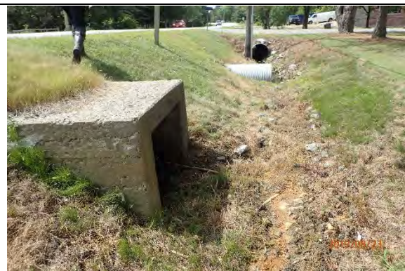
An abandoned box culvert was observed east of the current CSP crossing.
