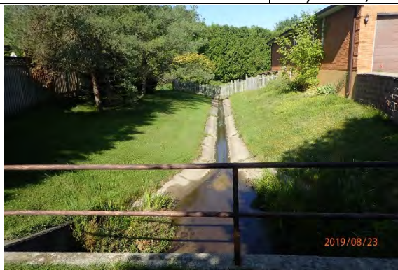
The reach was a concrete channel downstream of Archibald Road.
