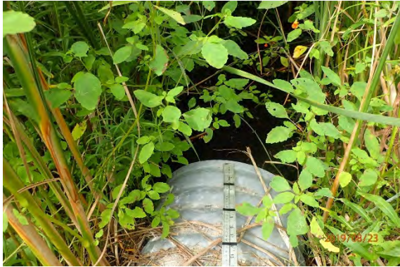
Photograph taken upstream of the crossing. The channel had cattails growing on the bed and grasses on the banks.
