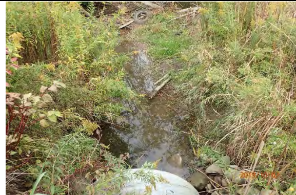
Photograph taken facing downstream of Lloydtown/Aurora Road. Minor bank erosion was noted on both sides of the channel to the confluence.
