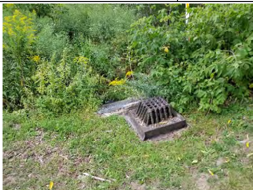
Reach HN4-4 flowed into a catch basin. Reach HN4-3 is piped to downstream of HWY 27.
