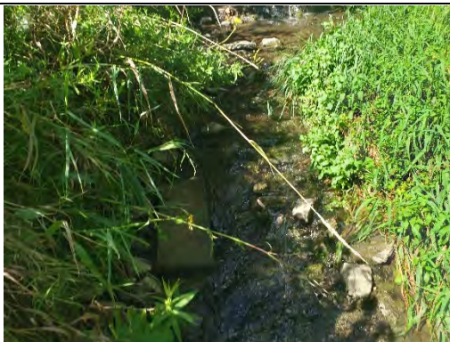
Photograph taken facing upstream. Bank undercutting measured to 0.05 m.
