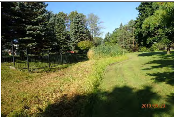
Downstream Cutting Crescent. Poorly defined swale feature which was heavily encroached with grasses. Note cattails further downstream.
