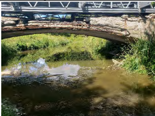
Newly renovated bridge crossing at King Vaughan Road. Photograph is looking upstream.
