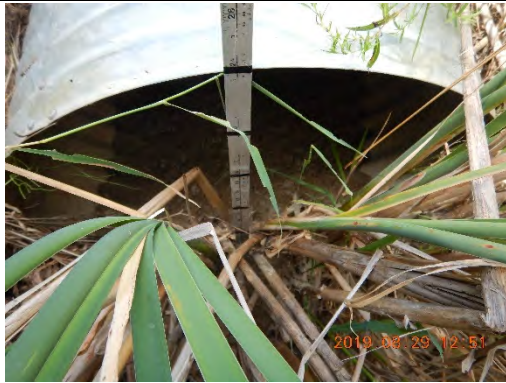
CSP downstream of 8 th Concession. The channel was dry at the time of assessment.
