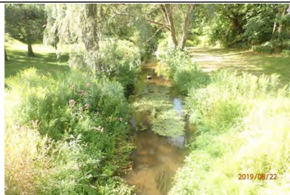
Sedimentation and pooling upstream of the crossing that was caused by the weir structure downstream of Rebellion Way.
