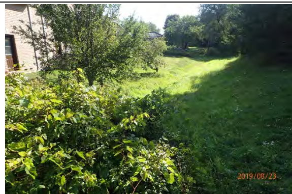
Upstream of Archibald Road. The swale continued to be poorly defined and heavily encroached with grasses.
