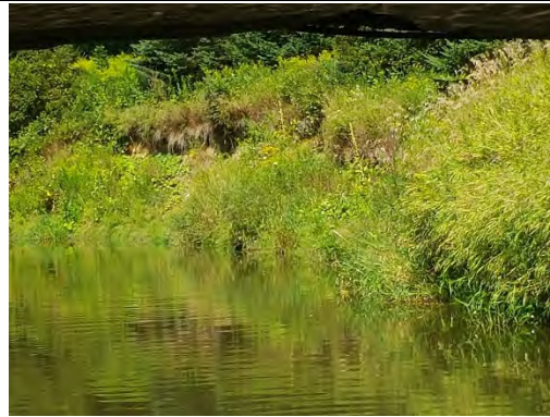
Photograph looking upstream at a vegetated bank where a slump had previously occurred.
