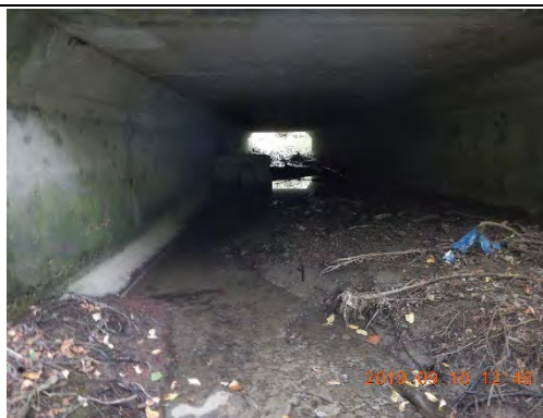
Culvert under Martin Street. There were no bridge footings exposed.
