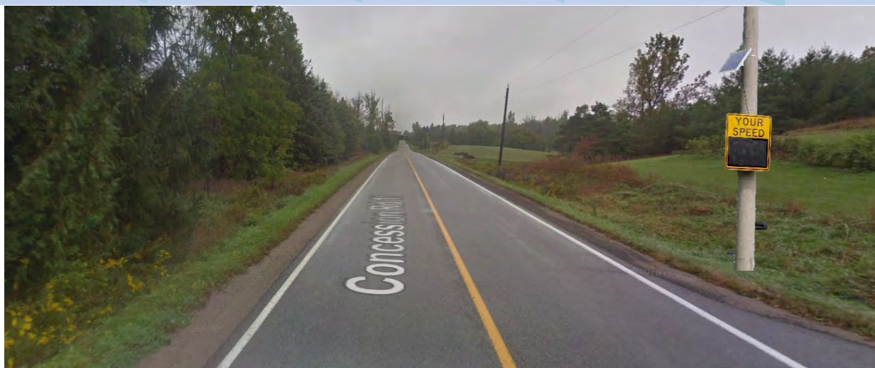
Figure 3-5: Rural Roadway with Pavement Markings and Speed Radar Sign
