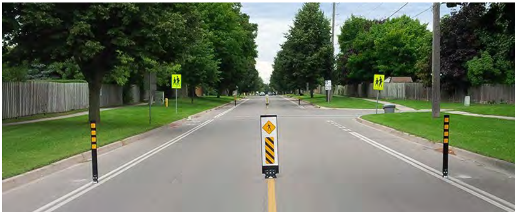
Figure 3-1: Typical Flexible Bollard Installation
