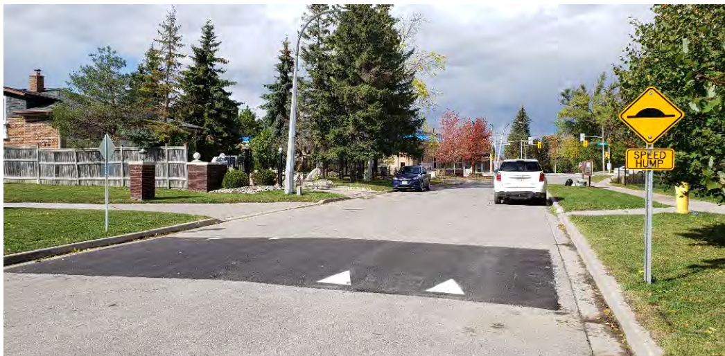
Figure 3-3 Speed Hump Installation Example on Banner Lane
